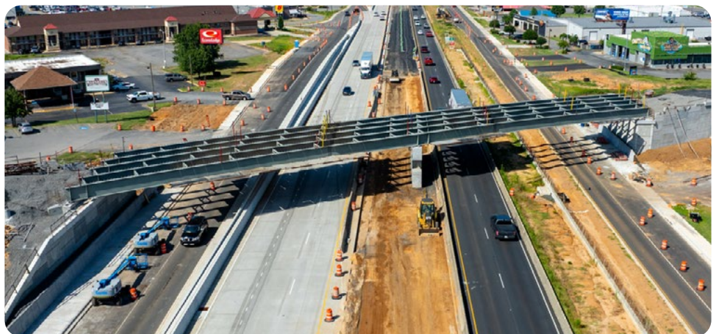
Gregory Street Overpass - Bridge Beam Installation
