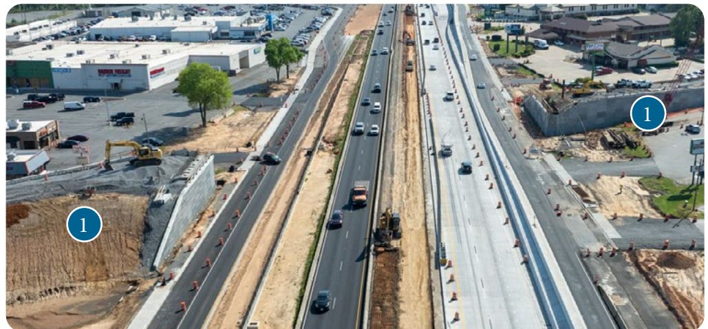
1 Gregory Street Overpass Construction
