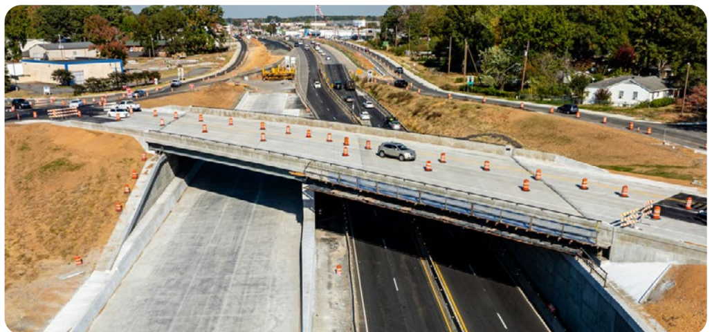
New N. James Street Bridge Opened October 2024
