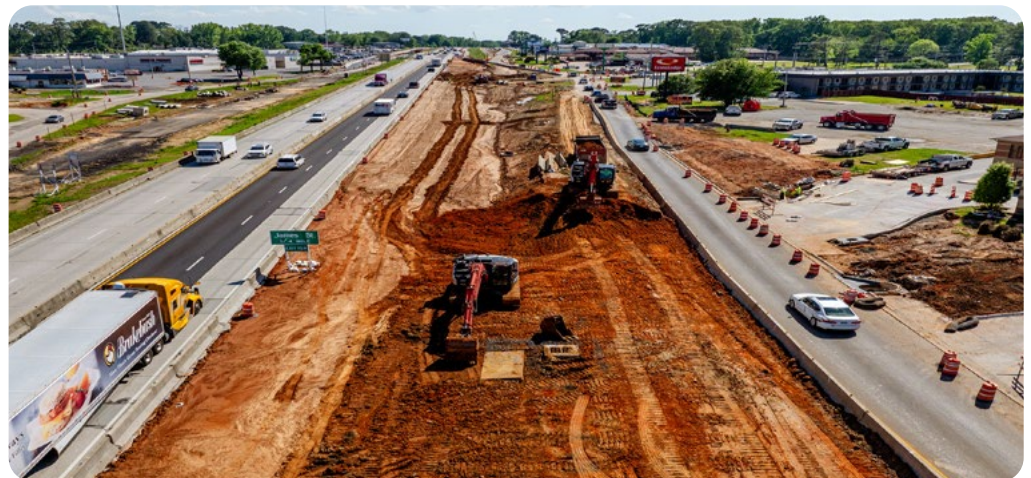
Highway 67 new southbound lanes being constructed
